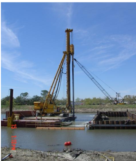
Photograph 3. Wet DMM operations from barge at Orleans Avenue Canal, New Orleans (Bruce et al., 2012).
