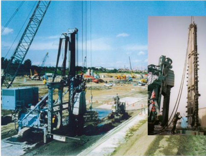
Photograph 6. TRD Method equipment.
