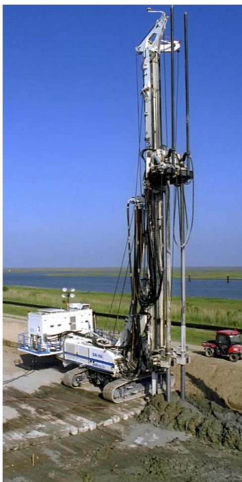
Photograph 4. Double axis Soilmec deep mixing machine at LPV 111, Louisiana.
